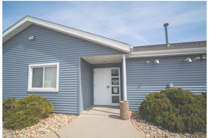
Clinic Administrative Building
